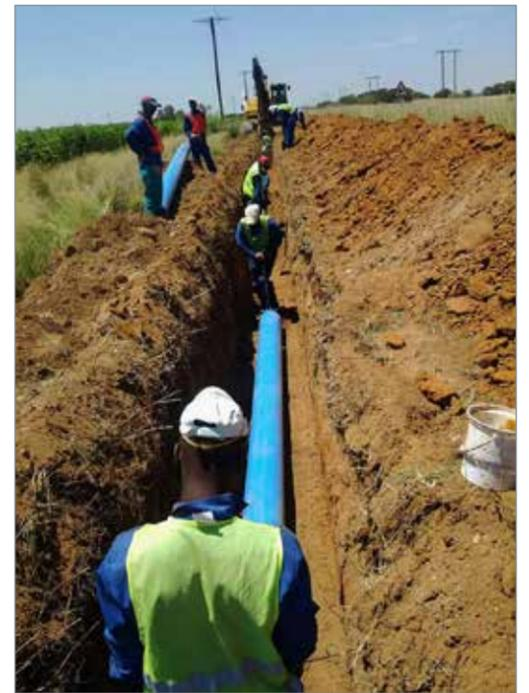
correctly and meet international standards, these pipes are cheaper, quicker and easier to install, do not rust, the joints are leak-proof (if installed correctly) and have lower failure rates than pipes made from alternative materials," Smit says.
